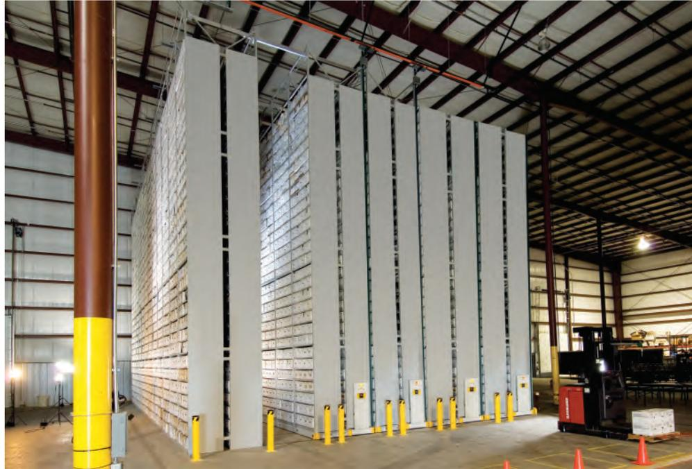
Stoffel and Spacesaver integrate Very Narrow Aisle trucks into storage system.
